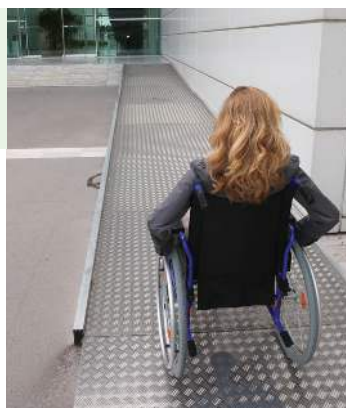
Figure 19.2 Wheelchair access ramp
